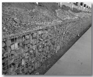
This gabion retaining wall is made of recycled concrete in baskets.
