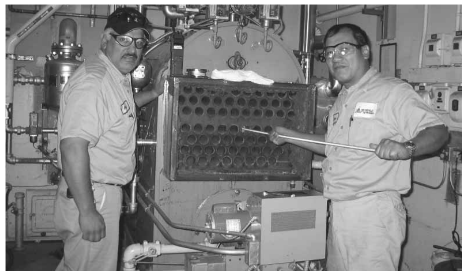
Efren Callenta (L) has maintained Moffett's boilers and Facilities Control Management System for 11 years. Andy Angeles has worked on the energy management system for 18 years. Here, they're working together to inspect all the safety parameters of the boiler and do the annual cleaning. Efren did similar work when he was in the Navy; Andy started at Moffett as an apprentice.
